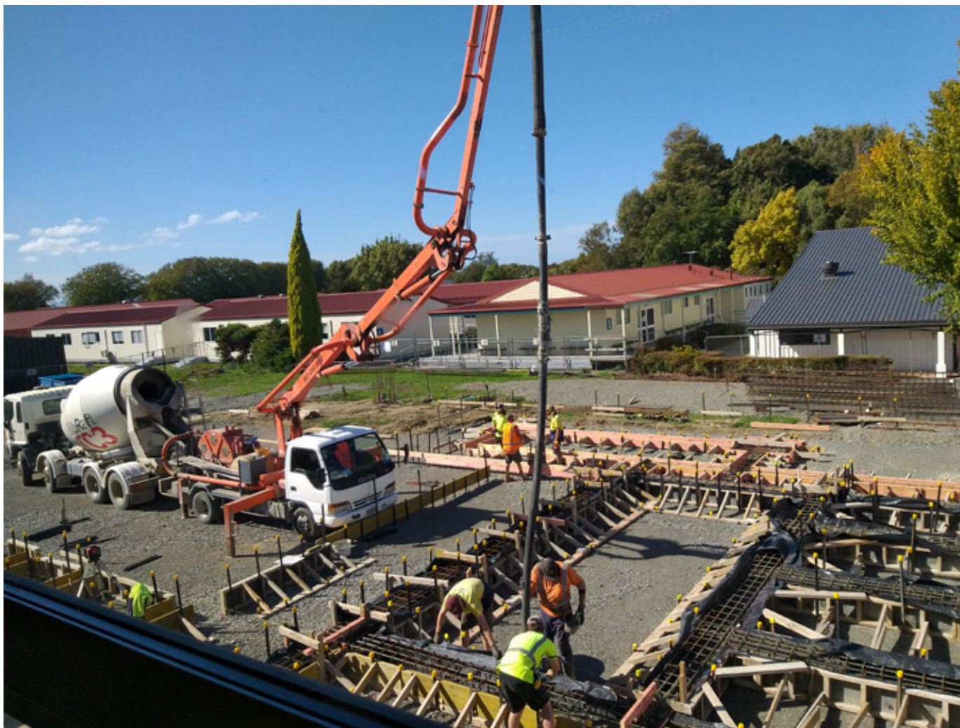
April 2021 - Concrete floor is poured
