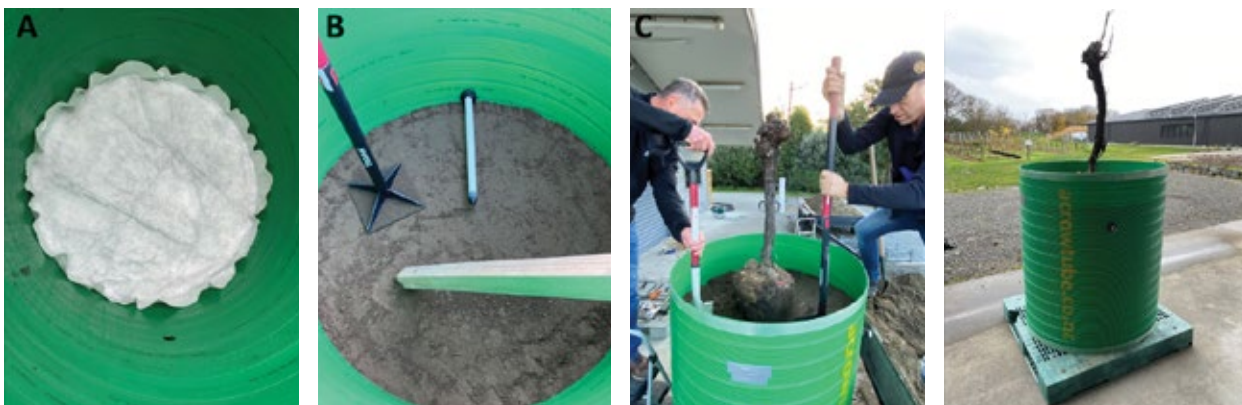
Prototype grapevine planter construction and filling.
